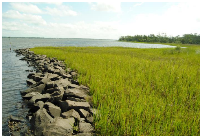
Hybrid living shoreline with rip rap. Image credit: Jesse baud, living shoreline , https://www.flickr.com/photos/151809992@N06/37911236174 , (CC0 1.0).
