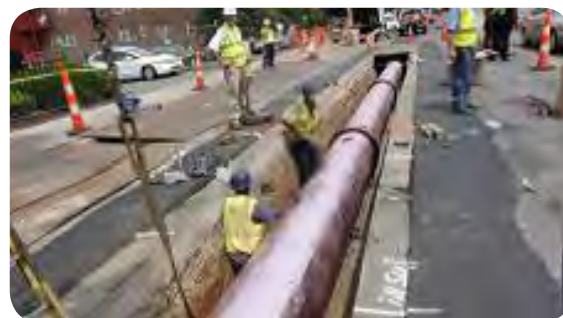
Water Main Installation Photo by DPH.
