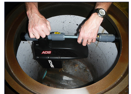
ECHO with installation bar mounted on manhole frame
