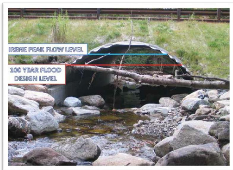
*Stream simulation design culvert at Jenny Coolidge Brook, installed in June 2010, showing height of 100-year design discharge in red and height of Tropical Storm Irene flood level in blue.<sup>14</sup> Photo credit: Brian Austin, Green Mountain National Forest*
