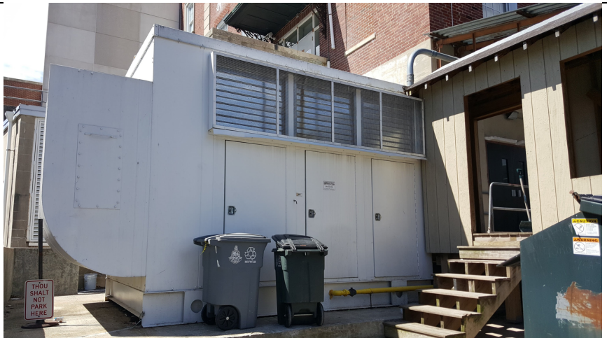
250kW natural gas-fired standby generator to supply main gym, locker rooms, cafeteria, kitchen, and auxiliary gym.
