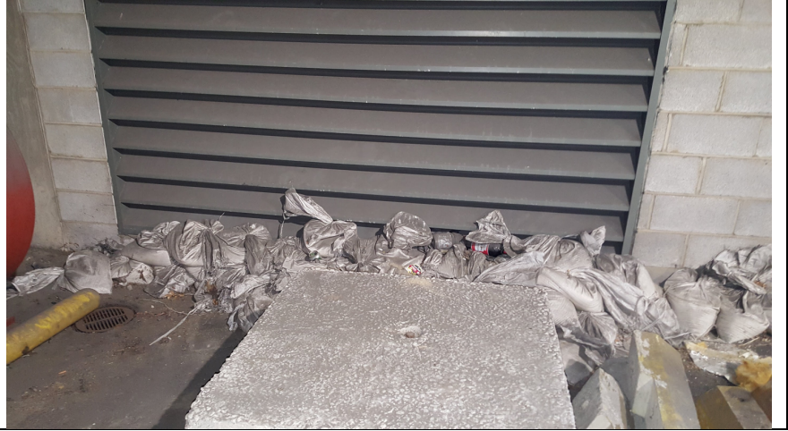
Sand bags at generator air intake in garage.
