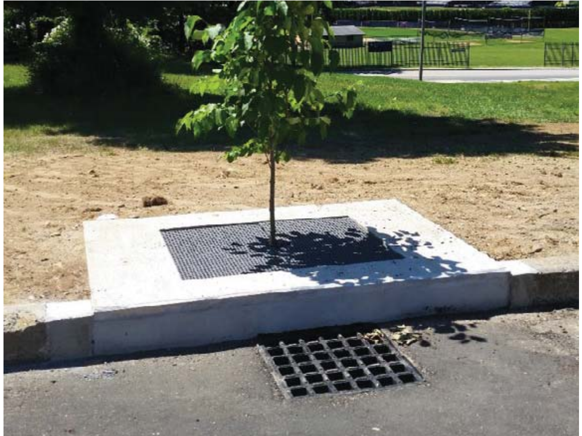
Stormwater Tree Box at UConn-Storrs. Courtesy of UConn CLEAR
