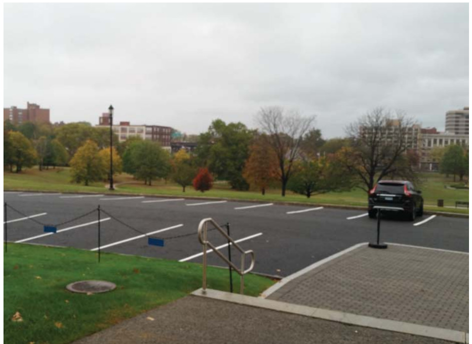
Porous asphalt parking lot and path with permeable pavers and pervious concrete on a rainy day at the CT State Capitol
