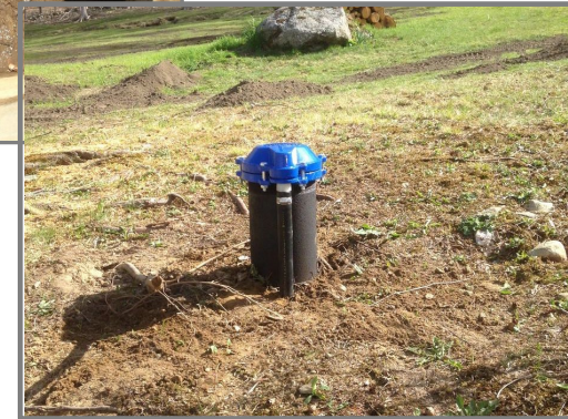
Well water casing extension - Oxford, CT Eastern Water Solutions
