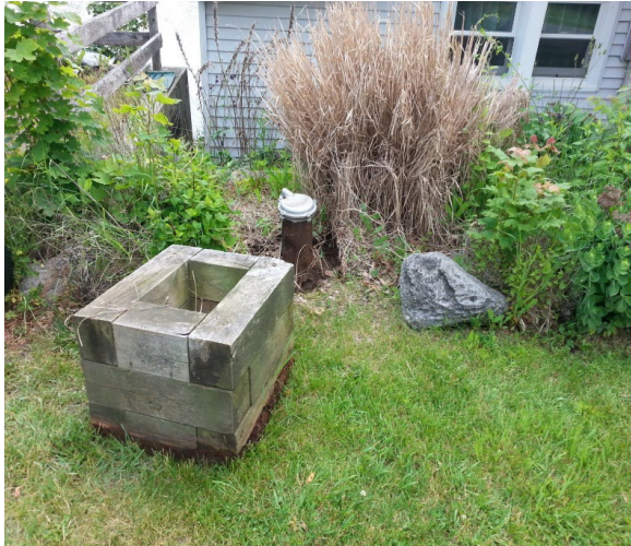
Wellhead located on Daniel Ave. in Guilford
