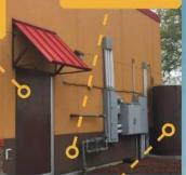
"Secure Tanks" to buried concrete bases or other anchors to resist floodwaters and avoid spillage of hazardous materials into the environment.
