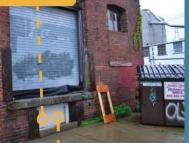
"Wet Floodproofing," such as louvered vents, could be installed in openings leading to basement or crawl space to improve the building's ability to withstand hydrostatic pressure caused by floodwaters.
