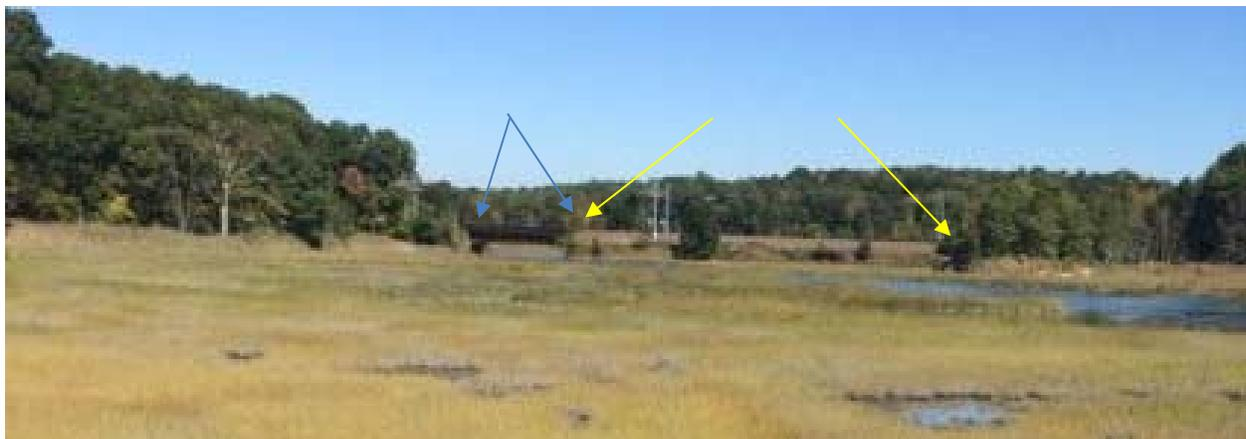
**Figure 2.** Photograph of the Amtrak railway causeway and bridge across Jarvis Creek marsh. The blue arrows indicate the width of the bridge and the yellow arrows show the raised causeway.
